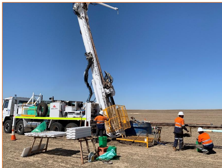
Diamond Drilling at Cadoux HPA Project
