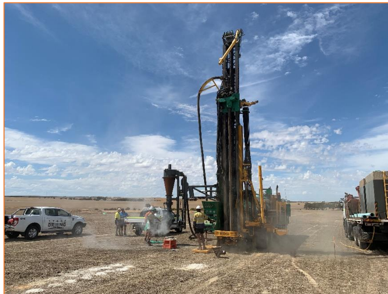
RC Drilling at Cadoux HPA Project
