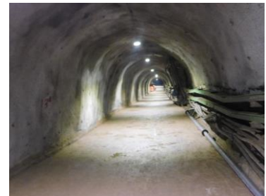
Access drive at the 190L of the Sino-Lao potash project
