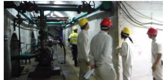
Images of Sino-Lao underground inspection
