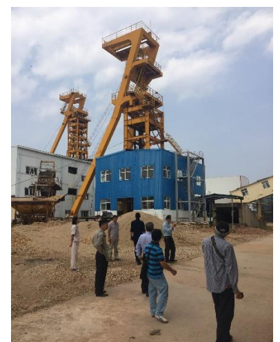
Image of Main and Auxiliary shafts at Sino-Lao Potash processing facility
