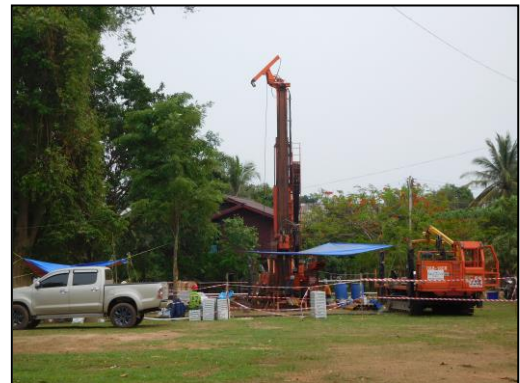
Drilling in the village square at Natan Project, Laos
