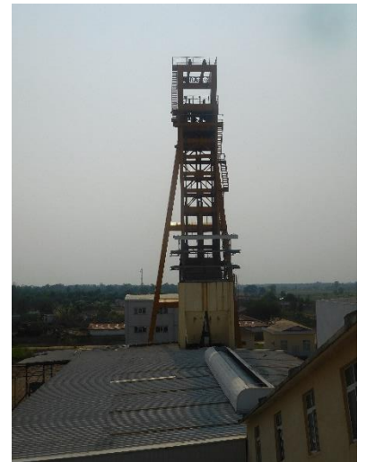
Sino-Lao Potash Project – view of auxiliary access shaft.
