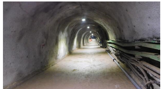
Sino-Lao Potash Project – view of 200 level access drive.
