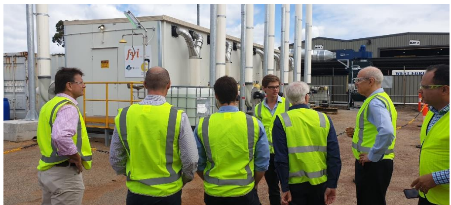
A tour group viewing the exterior of FYI’s HPA Pilot Plant prior to observing the continuous production
